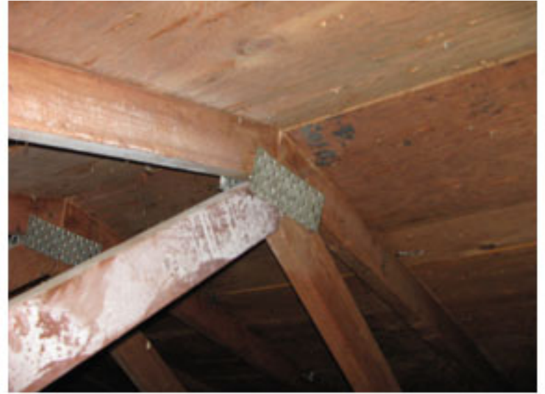
No notable attic decking stains from scuttle access
