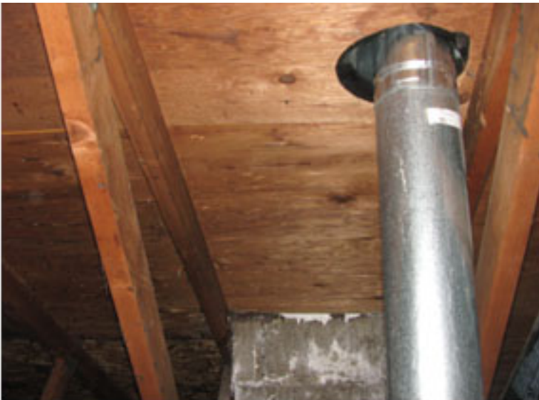
Roof decking from attic
