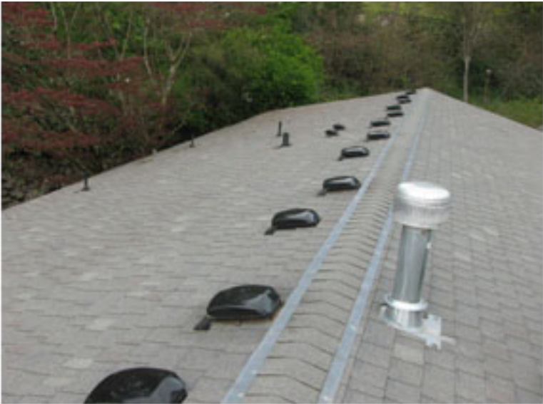
Lots of high roof vents
