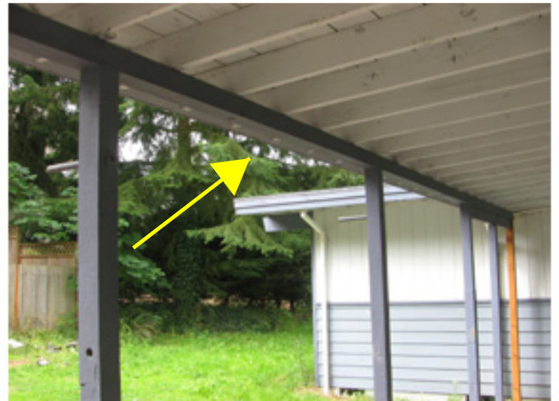
4x4 being used as a beam
