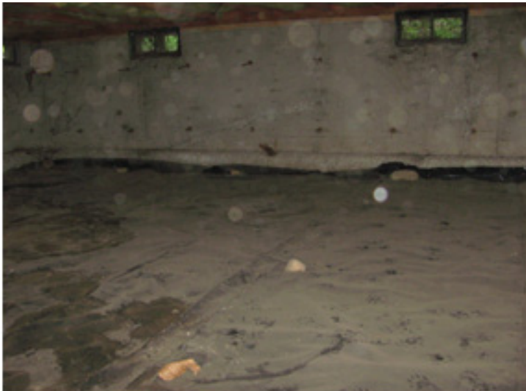
Crawlspace is dry
