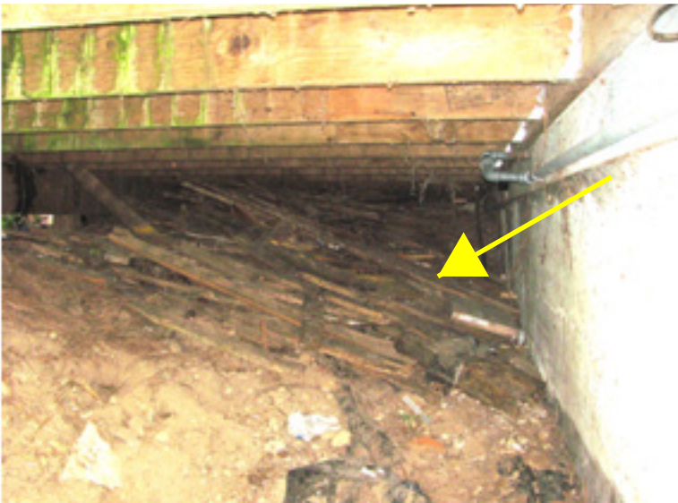
Remove wood cellulose debris from under the deck
