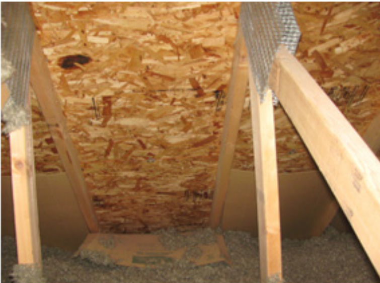
Roof decking and insolation in the south attic
