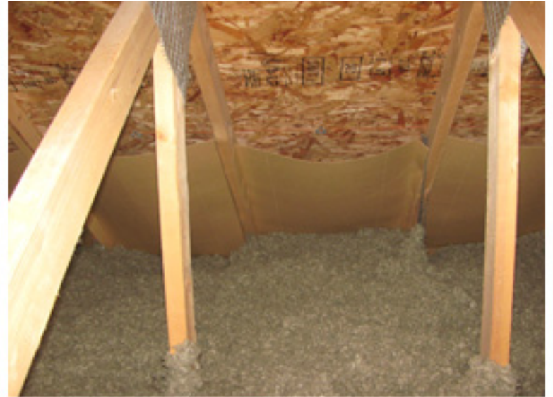
Roof decking and insolation in the north attic
