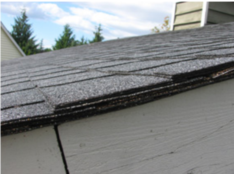
Two layers of roofing
