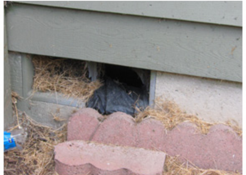
Repair foundation vent screen
