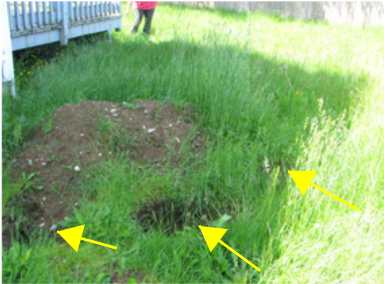
Septic access locations on NE exterior
