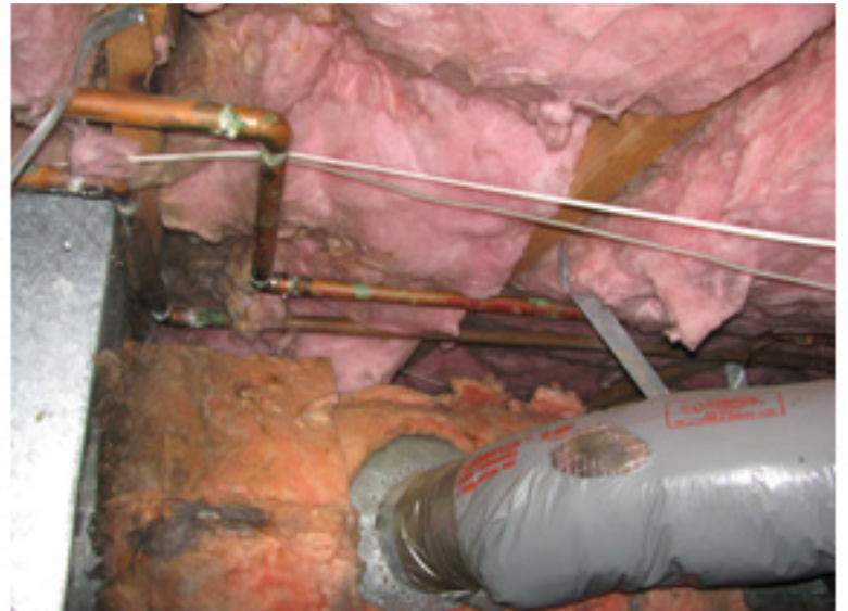
Insulate hot-cold pipes in the crawlspace
