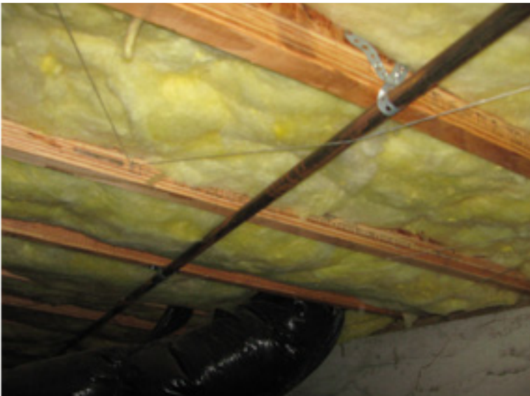
Insulate copper pipe in the crawlspace
