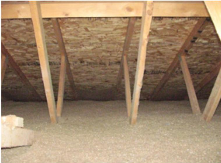
Cellulose insulation in attic. Roof decking is dry.
