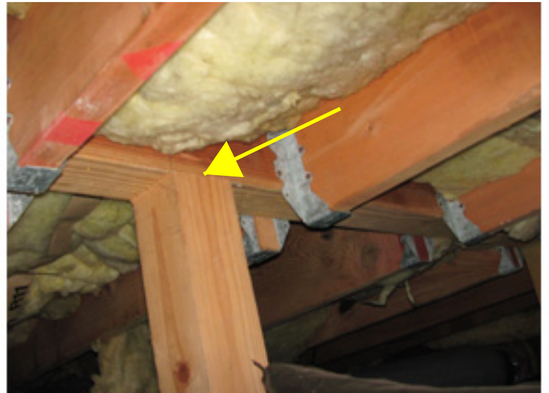
Gussets recommended on beam to post connections
