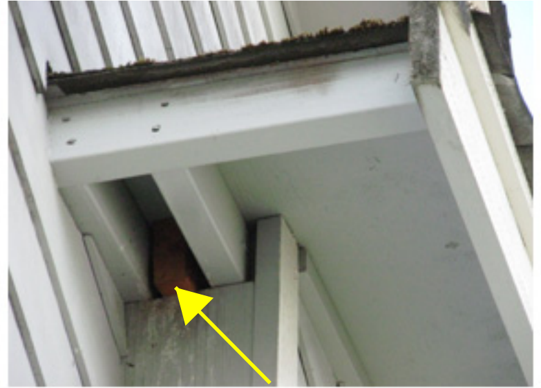
Fill ever hole with bird block or foam
