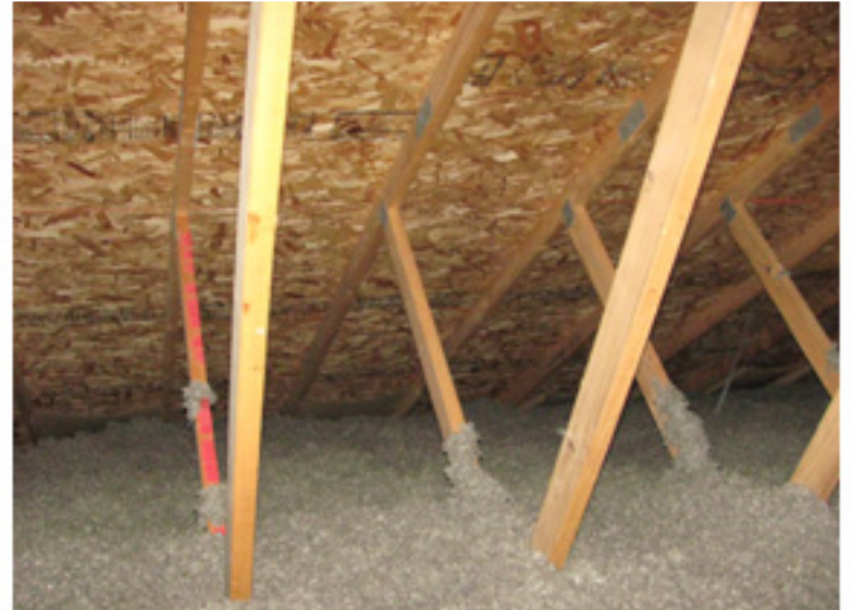
Roof decking in attic is dry - lots of insulation
