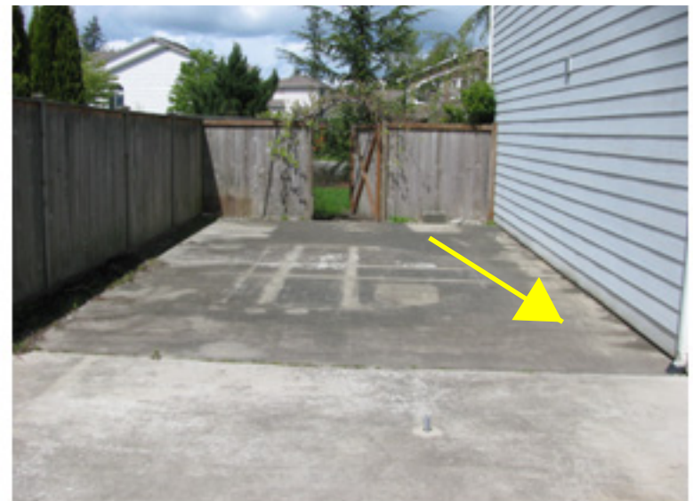
Concrete slab slopes to the house
