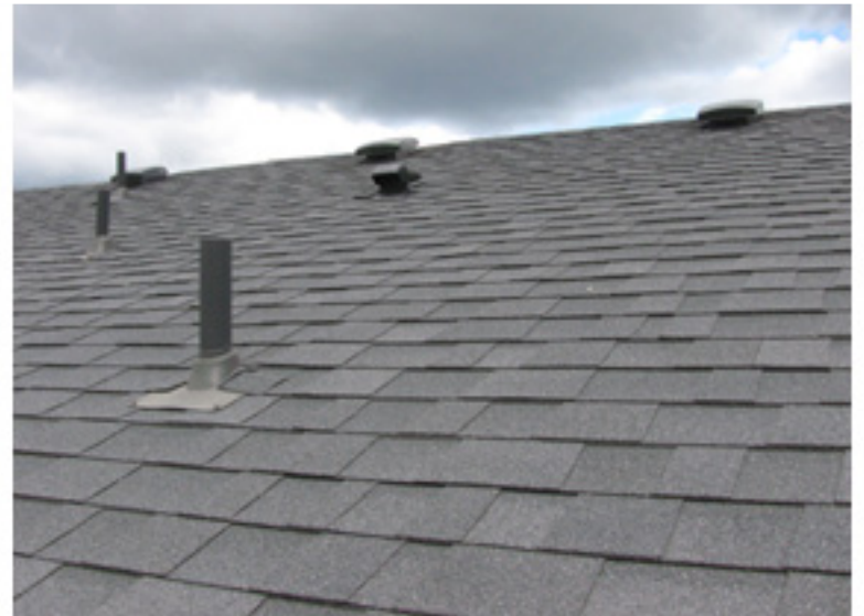
Roof is in good condition
