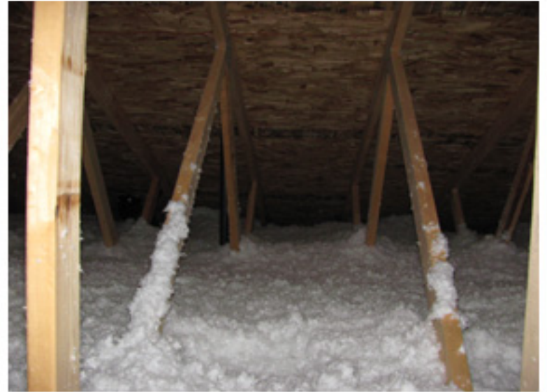
Lots of insulation in attic
