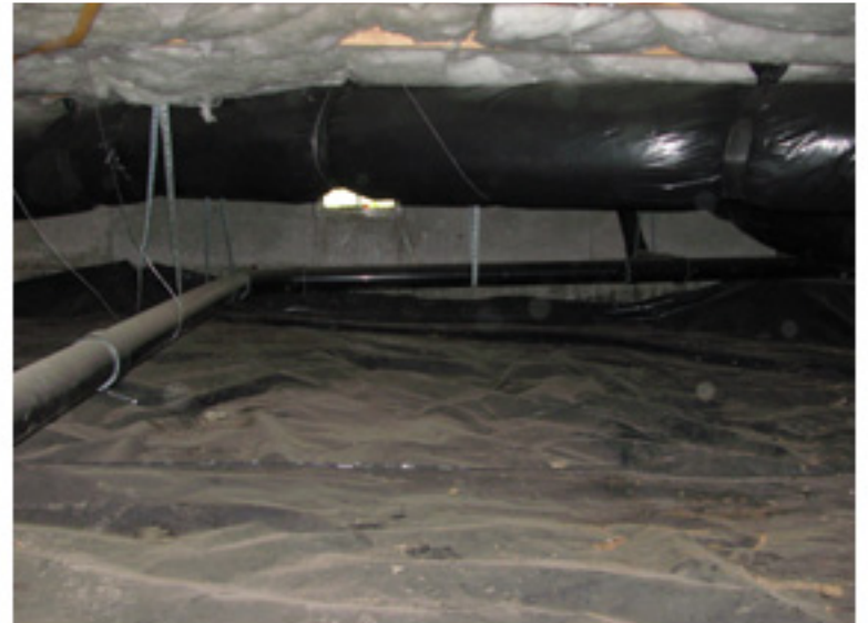
Crawlspace is dry
