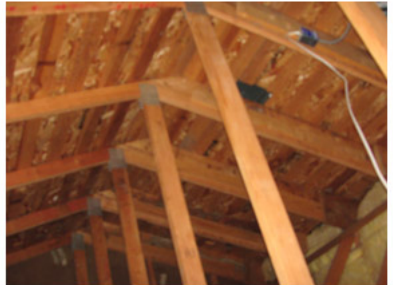
Attic decking is dry
