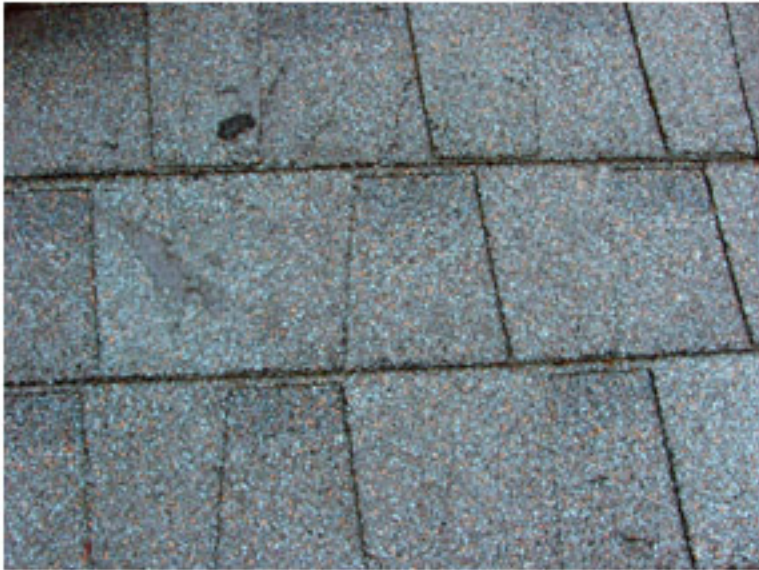
Roof shingles close
