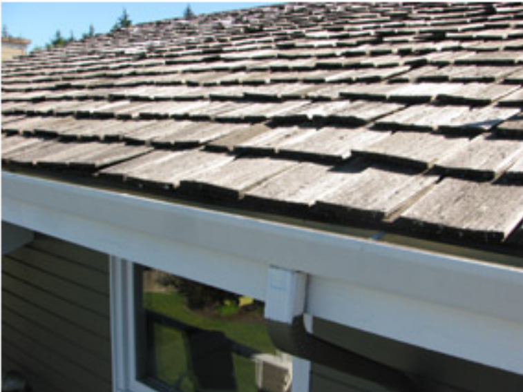
Back side roof
