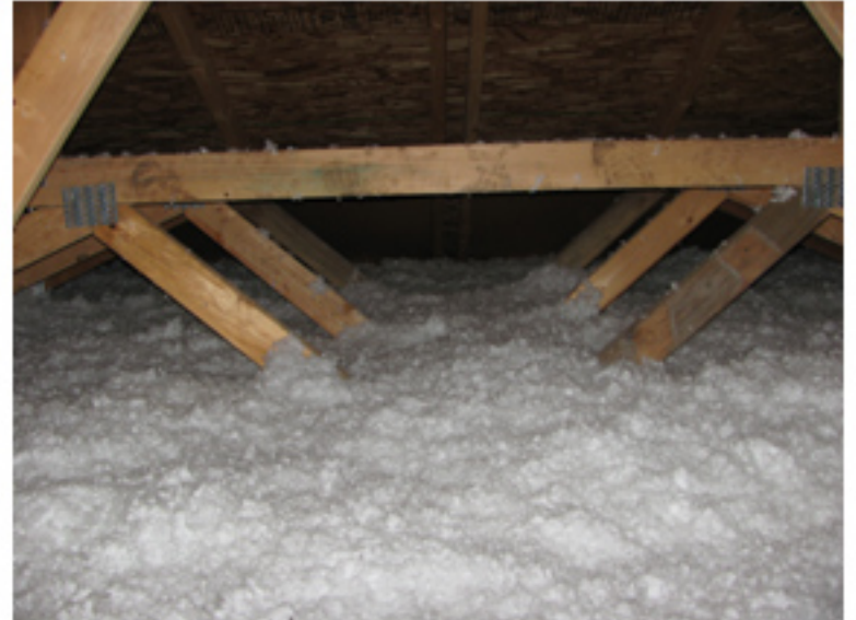
Lots of insulation in attic
