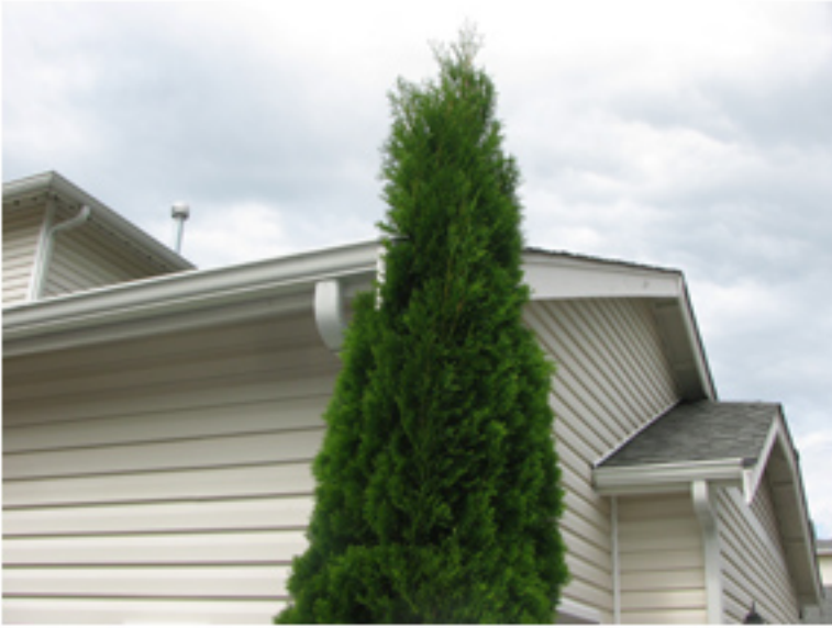
Trim vegetation away from the house
