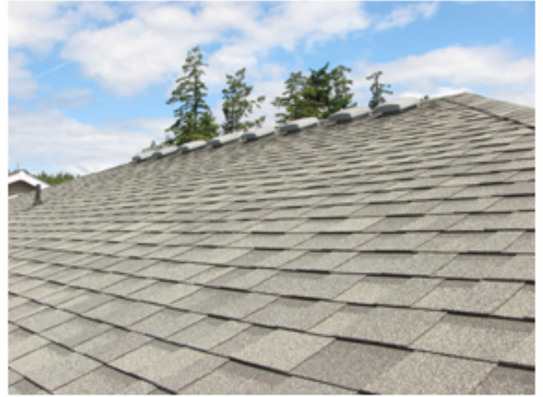
Lots of high roof vents. Good
