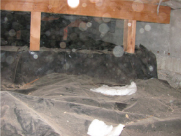
Crawlspace is dry
