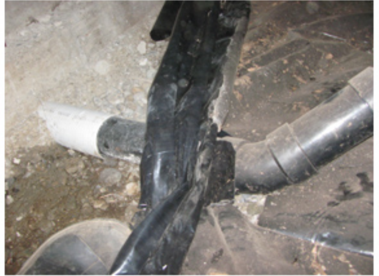
Positive sewer connection in crawlspace. OK
